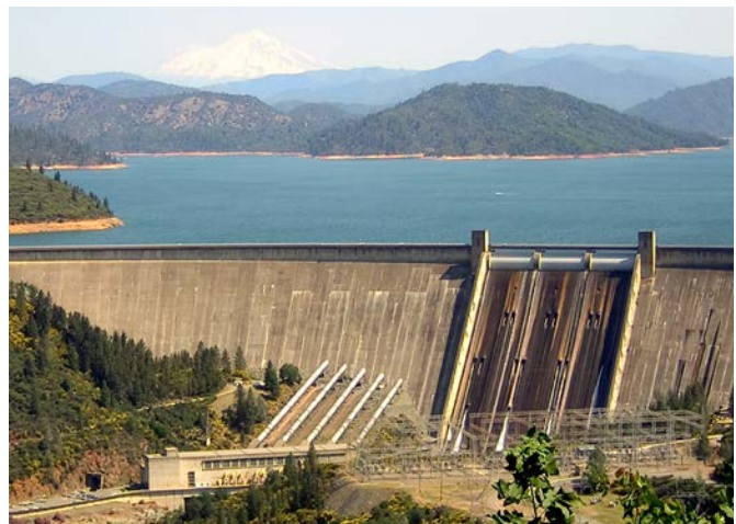
Shasta Dam, California
